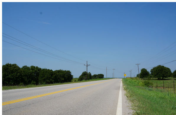
Figure 8. Two-lane rural road with no shoulders, Osage County, OK. Source: INCOG
