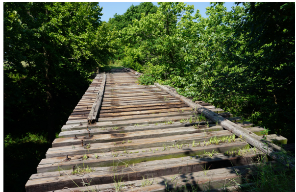
Figure 13. Former railroad bridge over Bird Creek, Avant, OK. Source: INCOG
