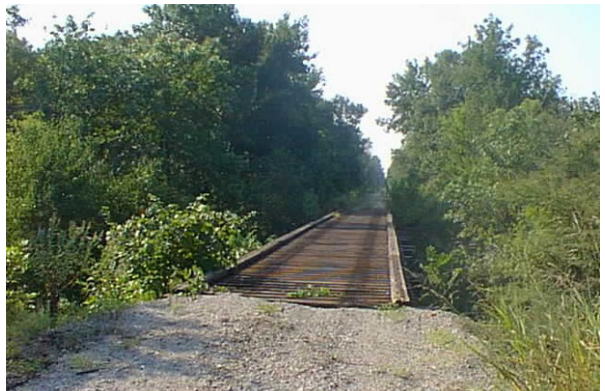
Figure 18. Former railroad bridge over Bird Creek, Avant, OK. Source: INCOG
