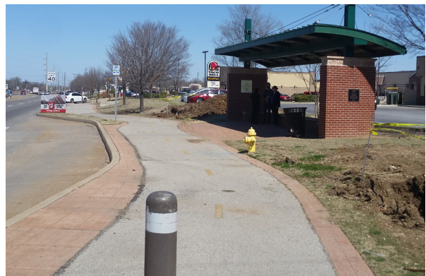
Figure 2. Sidepath on Peoria Avenue, Tulsa, OK Source: INCOG
